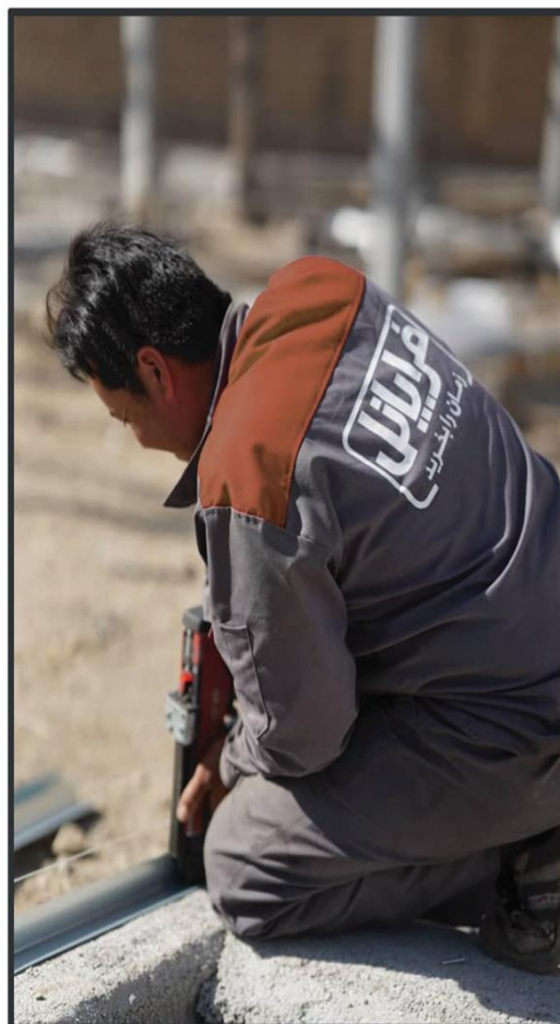
Installation of a runners on the floor and on concrete. 1
